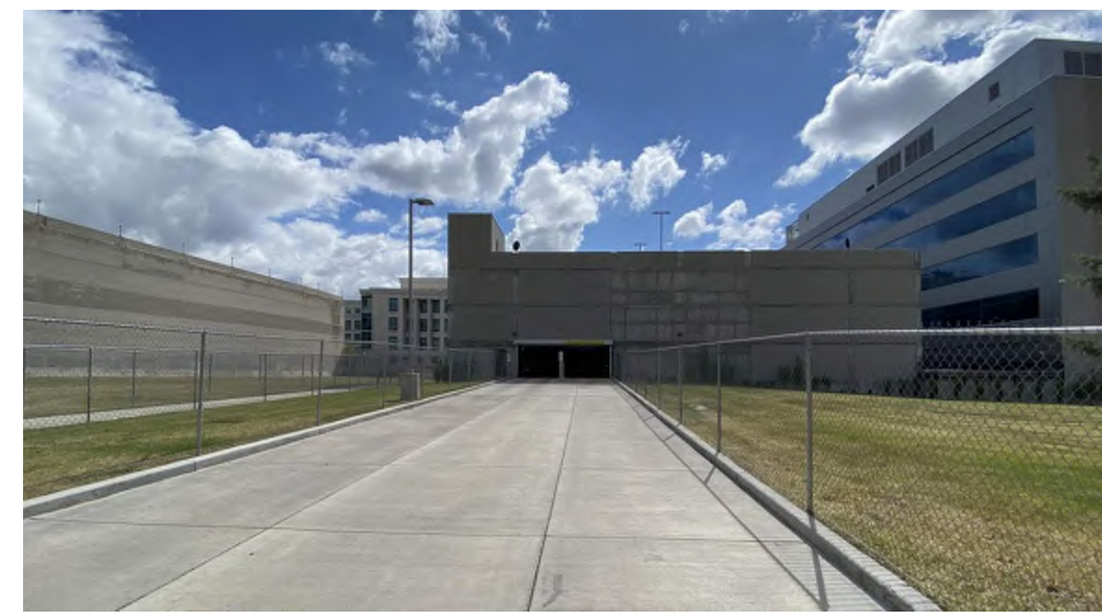
16. District Attorney Parking Structure
