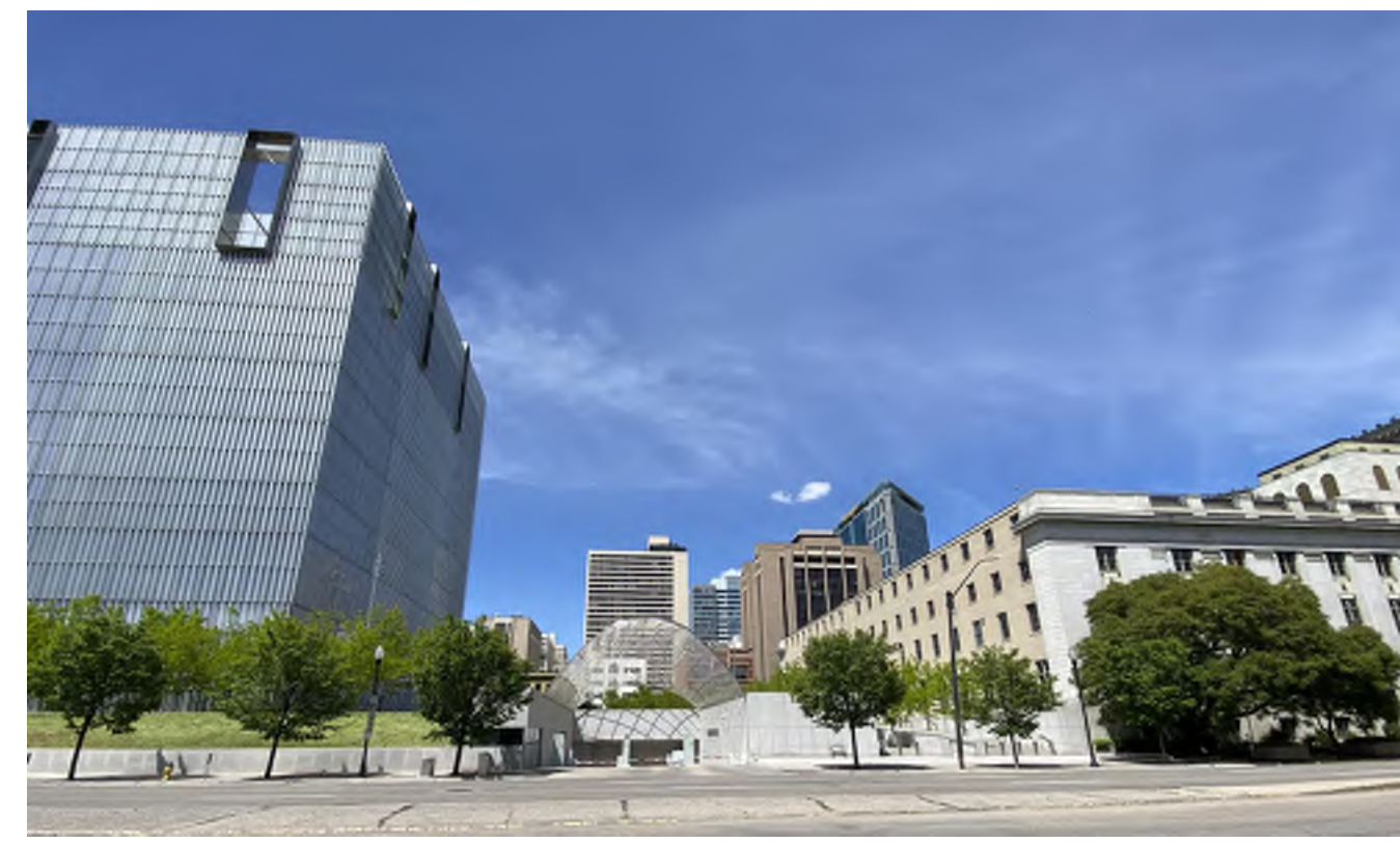
2. US District Court Parking
