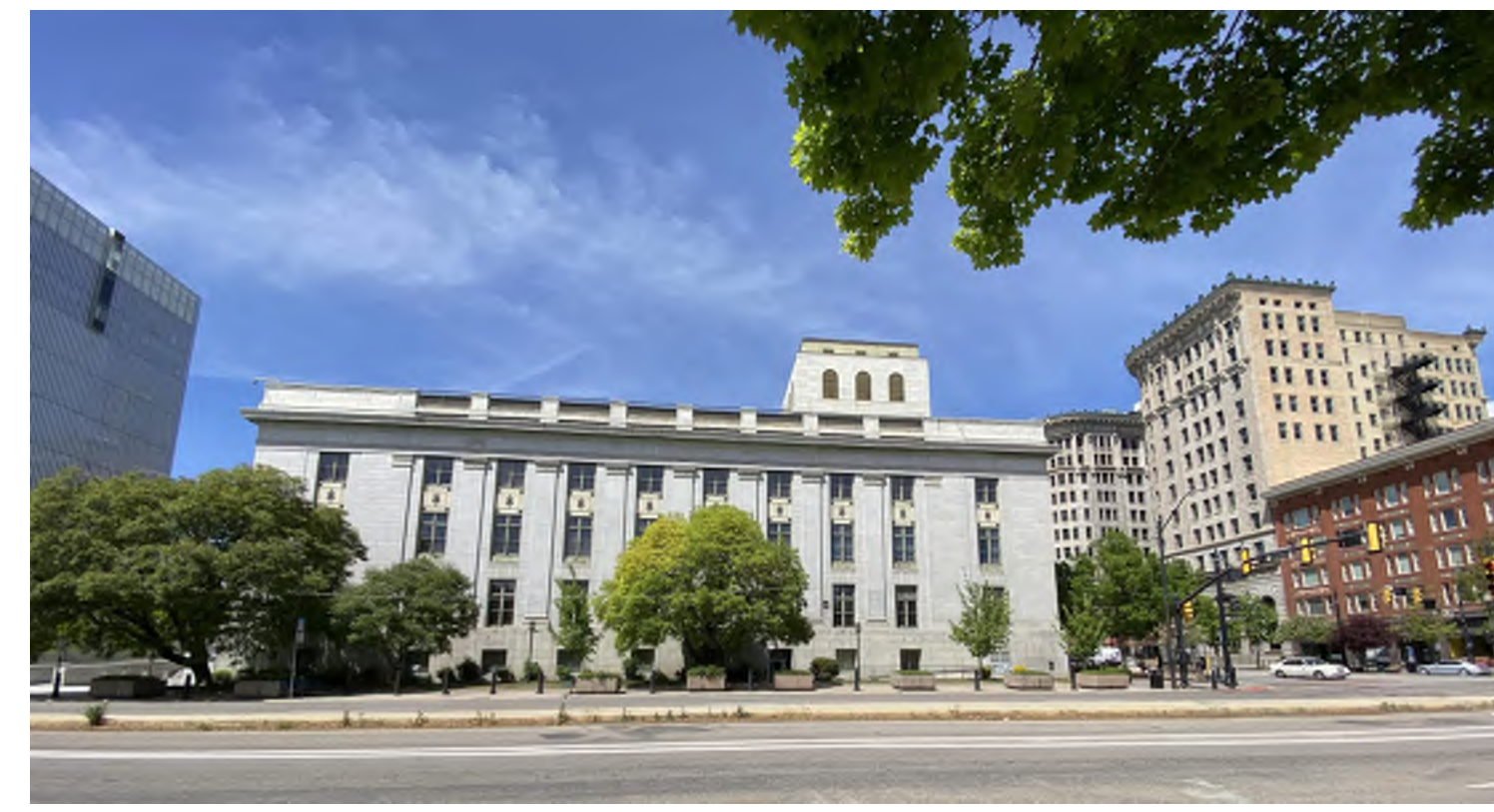
3. US District Court Parking
